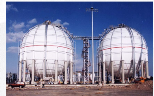
The Largest LPG tank in Asia, size: 8,000 m 3
