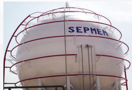
First double-shell tank in China
