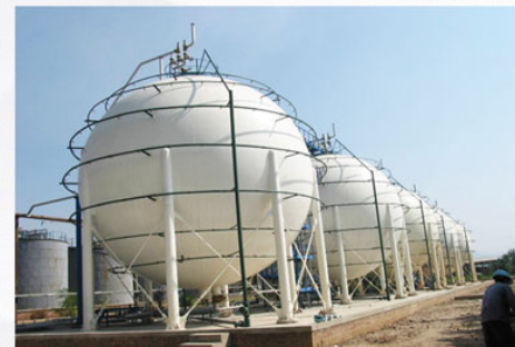
The largest ethylene spherical tank farm in China, size: 3,000 m 3
