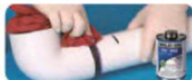
12. Remove the excess cement from the pipe and fitting 擦拭掉多余胶粘剂
