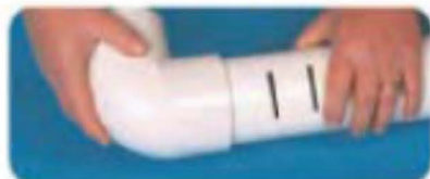
4. A dry fit "slop" test and mark this distance 干插测试, 划涂胶线
