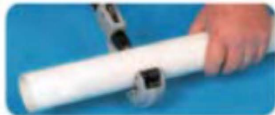
1. Cut pipe as square as possible 垂直切割管道
