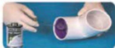
5. Apply the primer to fitting first 预粘胶先涂抹管件
