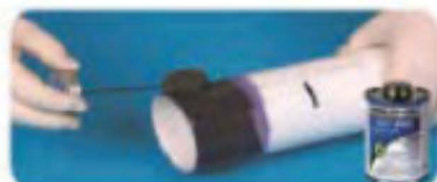
8. Apply the appropriate cement to the pipe 胶粘剂涂抹管道
