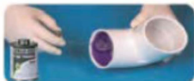
7. Apply a second application of primer to the fitting socket 再次涂抹管件
