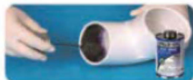
9. Apply the appropriate cement to the fitting 胶粘剂涂抹管件
